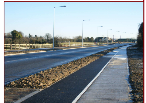
Distributor Roads & Associated Services, Balbriggan Co Dublin. (c. €10m)
